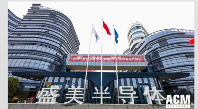
Lingang R&D and Production Center >1.4 million ft 2 (Lingang)
