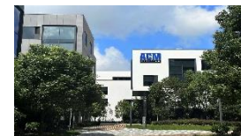
Shanghai R&D Center (Zhangjiang)
