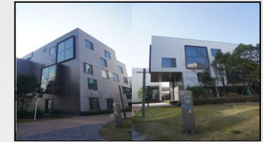
Shanghai R&D Center (Zhangjiang)
